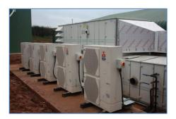
ABOVE: The building also runs an air handling unit for ventilation and emergency heating, along with five Mr Slim air conditioning units for additional heating and cooling when needed during the summer months.
