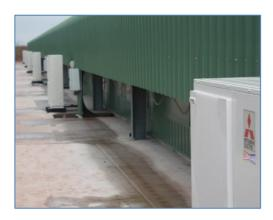
ABOVE: The six 14kW Ecodan units have proved much cheaper to run than the LPG heating on the other sheds.
