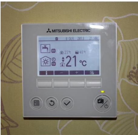
BELOW: Ecodan's intelligent, self-learning controls decide which heating system to use at any time to ensure the house is heated in the most economical way possible.
