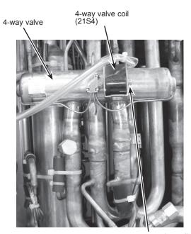
4-way valve coil fixing screw
