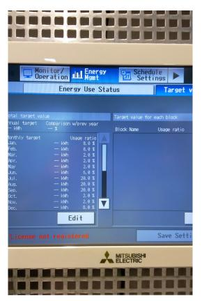
An advanced MelcoRemote control system has been installed to monitor the energy use of both the VRF and Hybrid VRF systems, along with the Ecodan heating units, lighting and extract fans within the building.
