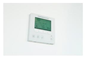
The new system is regulated using PAR-30MAA-J remote controllers which are simple and easy to operate.
