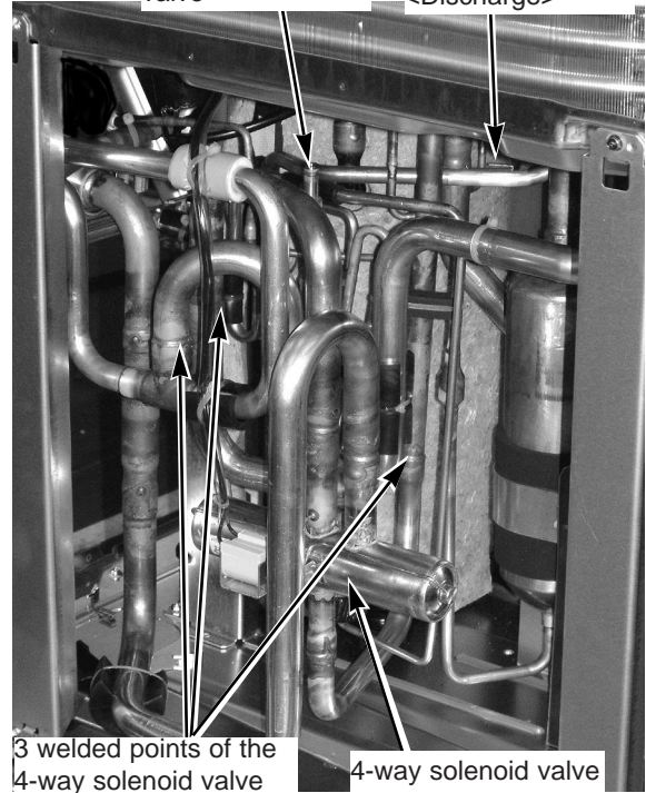
Photo 10 Bypass solenoid valve Thermistor <Discharge>
