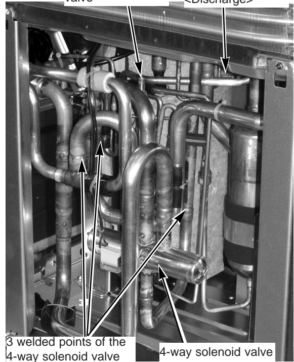
Photo 10 Bypass solenoid valve Thermistor <Discharge>
