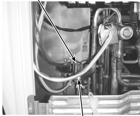
High pressure switch (63H)
