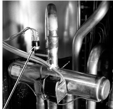
High pressure switch (63H)
