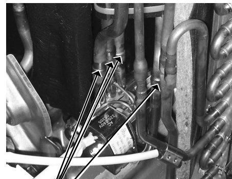
Welded parts of 4-way valve
