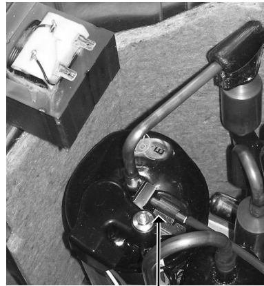
Discharge temperature thermistor
