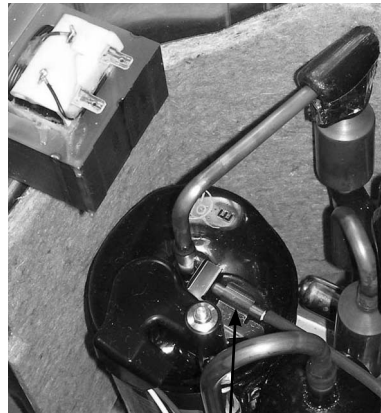
Discharge temperature thermistor
