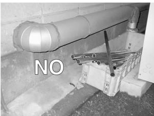
Store the pipes to be used indoors. (Warehouse at site or owner's warehouse) Storing them outdoors may cause dirt, waste, or water to infiltrate.
