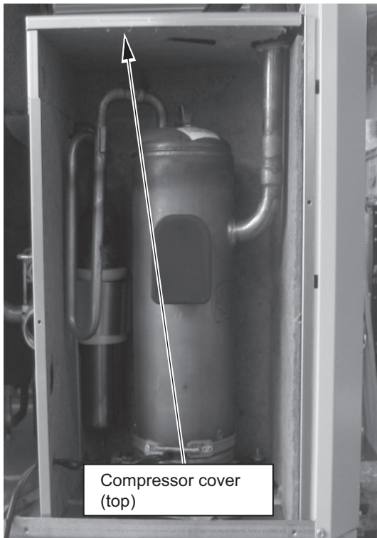
4. Remove the compressor cover (top).
