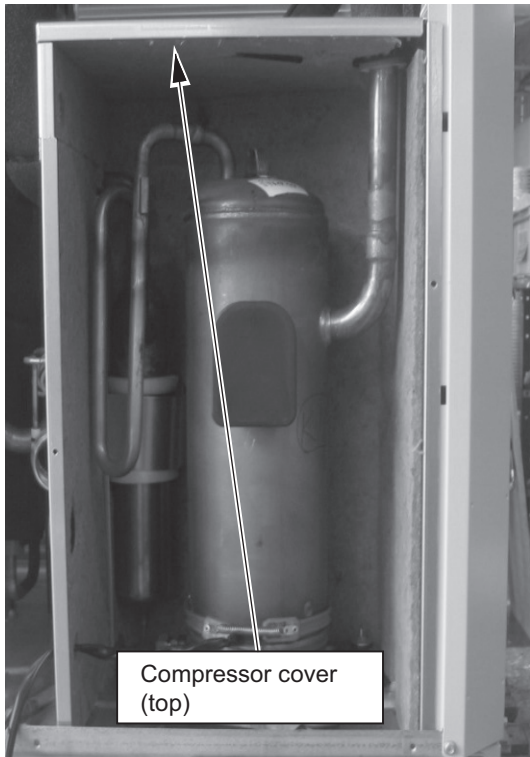
4. Remove the compressor cover (top).
