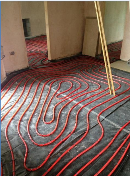
ABOVE: The home has underfloor heating throughout the ground floor and radiators in all first floor rooms.
