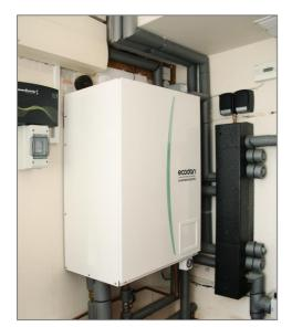
Above: The pre-plumbed and wired hydroboxhelps speed up installation and comes with simplified SD card commissioning.
