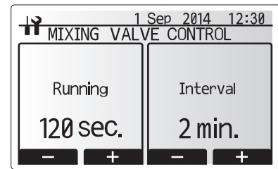
Mixing valve control setting screen
