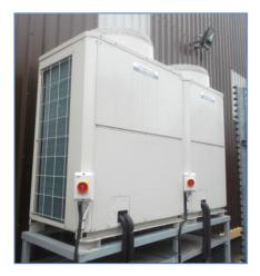
Modern air conditioning systems can often use the same piping as R22 units saving on installation time, as well as increasing performance and efficiency.
