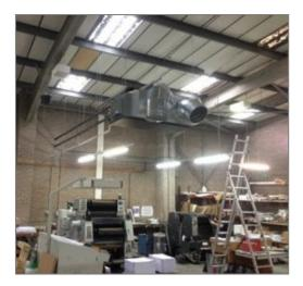
The solution was a Mr Slim ducted air conditioning system which is not only more energy efficient, it also evenly distributes heat down to the floor where it is needed. The old system just blew heat up to the ceiling.
