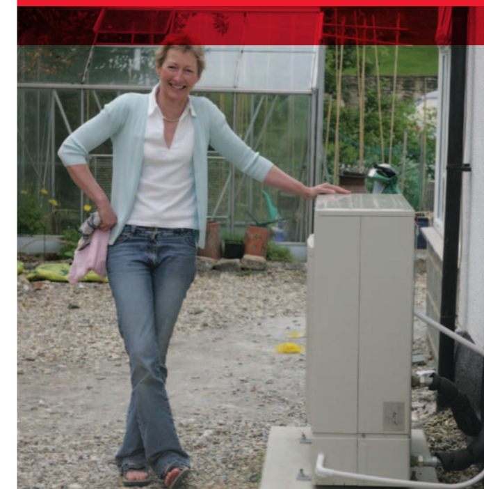
Heat pump solution for off-the-grid home
