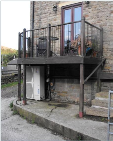
**ABOVE:** The 14kW Ecodan unit has been installed underneath the home's veranda.
