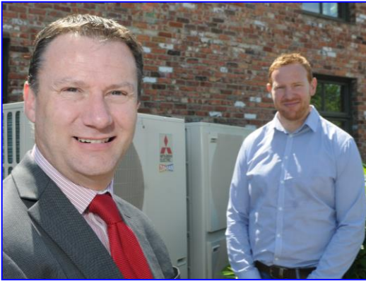
ABOVE: Groundwork's Andrew Watts (left) and Jason Oakes of Oakes Energy standing next to the four Ecodan air source heat pumps.
