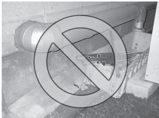
Store the piping materials indoors until they are ready to be installed (e.g., storage room on site or at the installer's premise). If left outdoors, dust, dirt, or moisture may infiltrate and contaminate the pipe, resulting in malfunctions.
