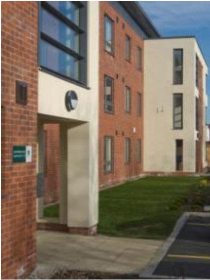
The stylish apartments benefit from low carbon renewable heating via a communal, underfloor system.
