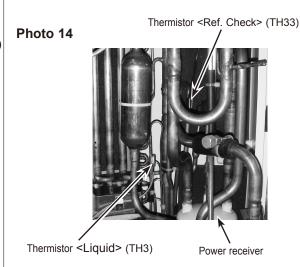
Note: The thermistor <Ref. check> (TH33) can be removed easily by removing the side panel (R).
