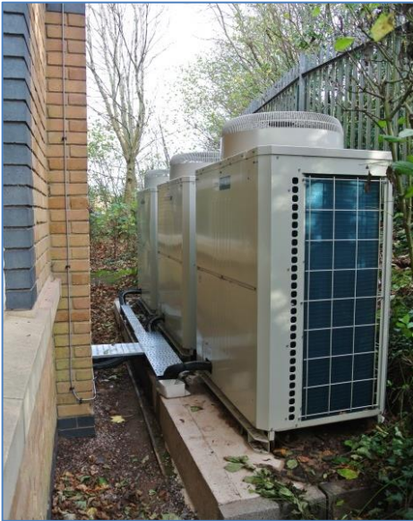
Hybrid VRF provides the same 2-pipe flexibility of traditional VRF, whilst delivering 4-pipe Chiller levels of comfort for occupants.
