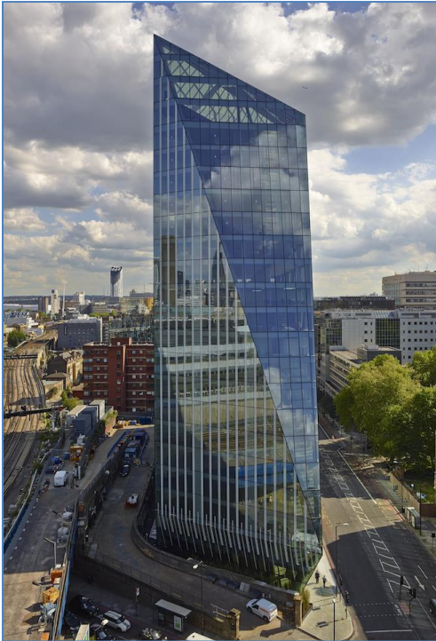
The new Pret a Manger store in the iconic building needed a sustainable, energy efficient solution that delivers first class comfort.
