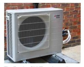
The Ecodan QUHZ outdoor unit sends renewable heat energy, harvested from the air to a thermal store, which then delivers hot water as required.
