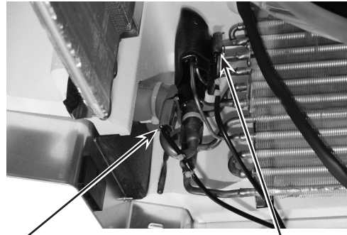
Condenser/evaporator temperature thermistor (TH5)
