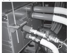
Install a non-return valve to prevent water in the water circuit flooding back to the water supply pipe, or remove the water supply hose after the air vent operation.
