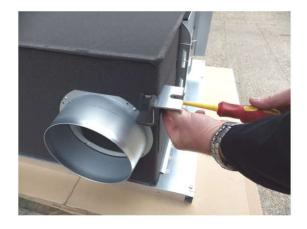
Align the back panel 5 to the Lossnay unit and fit using 3 x M6 X 12 set screws 11
