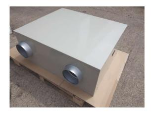
9 It is advised that the Lossnay unit and housing should be securely mounted on a suitable support to minimise vibration and movement and to ensure that the bottom of the air inlet spigot is at least 300mm above floor level.
