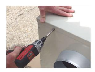
8 The Lossnay and weatherproof housing is now complete for final installation.
