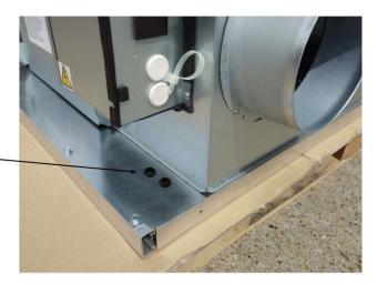
Remove the transport / hanging brackets from the Lossnay unit.
