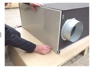
Align the OA & EA panel 4 to the Lossnay unit and fit using 3 x M6 X 12 set screws 11 and screw to the back and door panels using 4 x M4 X 25 set screws 9 and 4 x nylon washers 10
