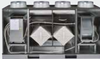
Removal of the front panels
