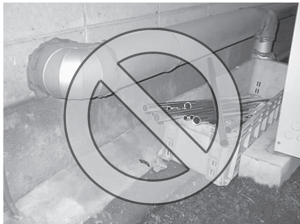
Store the pipes to be used indoors. (Warehouse at site or owner's warehouse)
