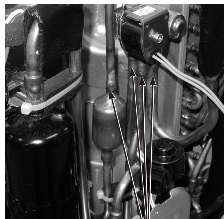
Brazed parts of 4-way valve
