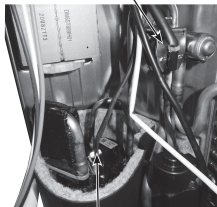
Discharge temperature thermistor
