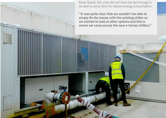
One of the Climaveneta chillers has now been replaced with six 180kW modular e-Series chillers - the first R32 units to be installed in the UK. These modern, inverter-driven chillers are specifically designed to modulate the cooling load to match the demands of the building.
