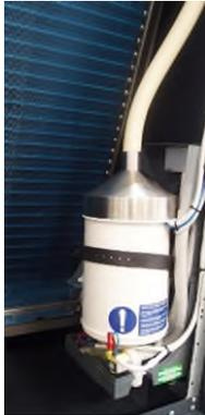
The humidifier's water intake connection is 3/4" G M – ISO 228/1 and it's water discharge connection is 32 mm M smooth pipe.
