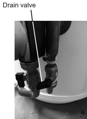
2. Turn off cold water supply to Heat Pump Cylinder. Drain down cylinder making sure Hot water outlet is isolated, connect hose to tail and secure. Run hose to drain.
