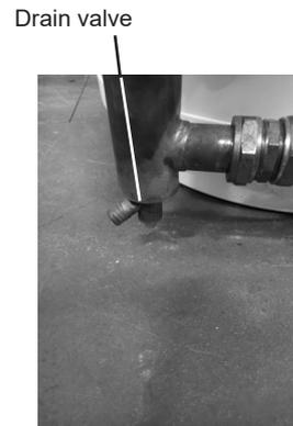
3. Drain down Heat Pump Primary fluid, ensuring it is disposed of in accordance with national environmental regulations.
