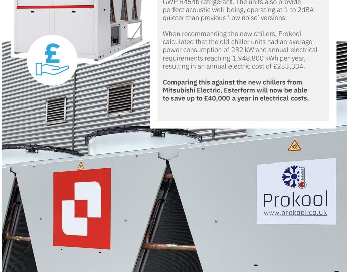
David Gawthrope at Prokool explained, "The new Mitsubishi Electric chillers use microchannel condensers and lower refrigerant R454B scroll compressors, both of which operate more efficiently than the technology in the previous chillers. As a result, Esterform will be able to bring down the electrical costs over time, which is a great benefit for the company".
