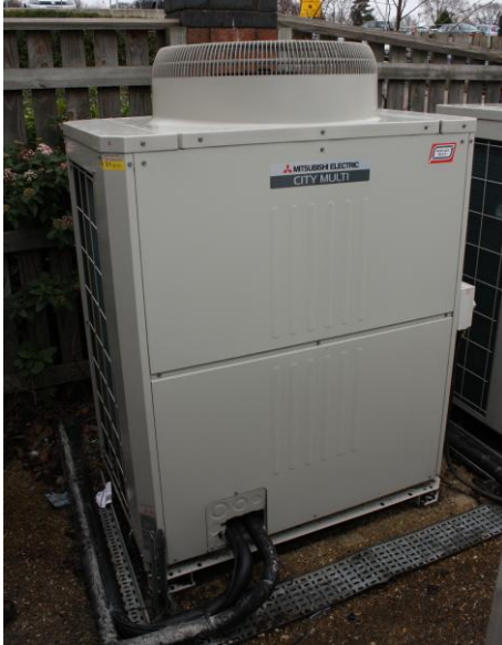
Mitsubishi Electric's City Multi YJM-A Replace Multi units were selected as the most cost-effective solution.
