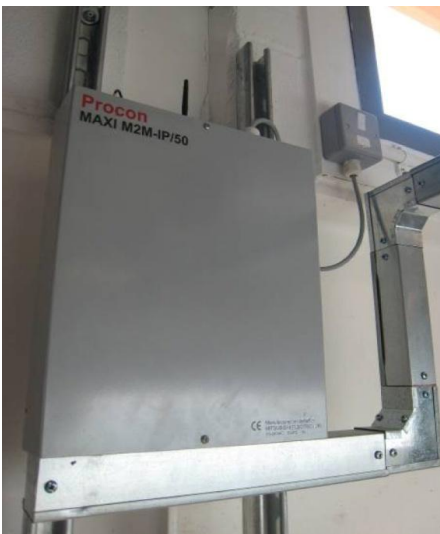
The entire system is monitored with Mitsubishi Electric's Maxi M2M-IP/50 controller, offering total control of efficiency and performance.
