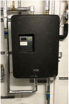
"The Regumaq decreases the temperature returning to the cylinder which in turn decreases the flow temperature going back to the QAHV,"
