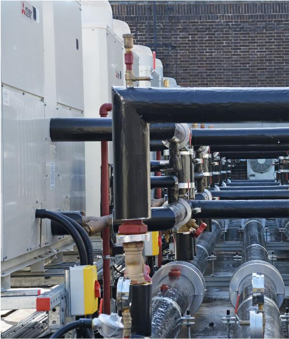
The CAHV heat pumps are ideally suited to this application as they offer a robust, low carbon system for the provision of sanitary hot water and space heating. The air source heat pumps can operate as a single system or, as in the case of the Civic Centre, form part of a multiple unit system, making it suitable for most commercial applications.
