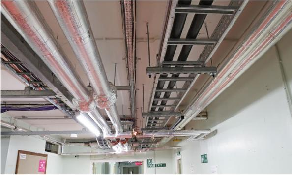
In addition to replacing the heating and hot water plant, RPS Group installed trace-heated primary circuit distribution LPHW (low temperature) pipework from the heat pumps to the existing plantroom.
