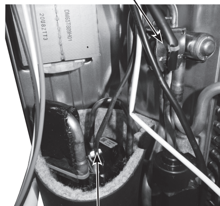
Discharge temperature thermistor
