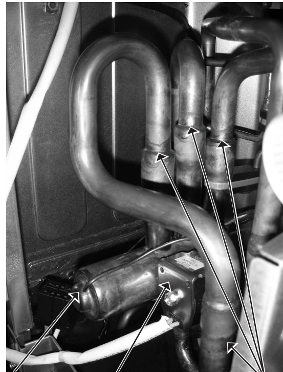
4-way valve R.V. coil Brazed parts of 4-way valve and pipes
