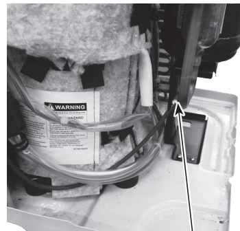
Thermistor <Discharge> (TH4)
