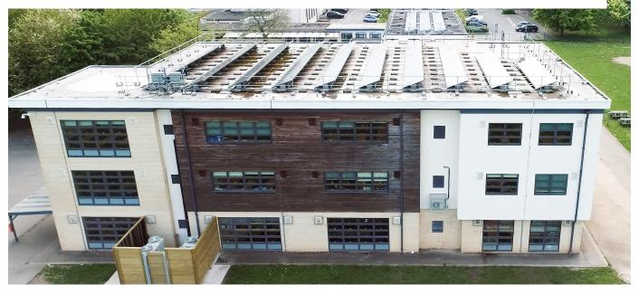
Although the CAHV units are very quiet at 64dBA, JM Renewables built an acoustic enclosure as the heat pumps are outside classroom windows.
