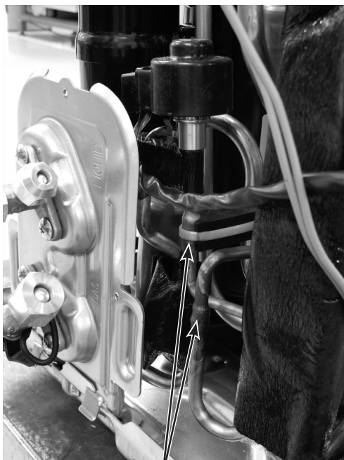
Brazed parts of the expansion valve
