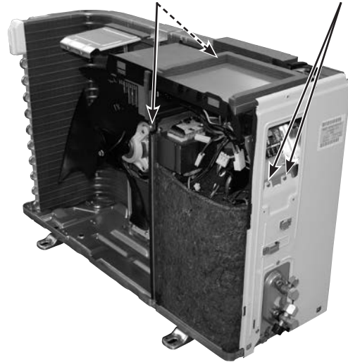
Photo 5 (Inverter assembly)
