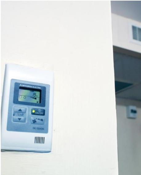
The temperature in unoccupied rooms is constantly monitored. Should it fall outside a pre-set range the unit automatically activates to cool or heat it.
